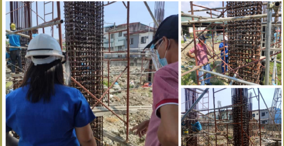
Status of construction of Casa de Silencio Retirement Home and Convention Center
